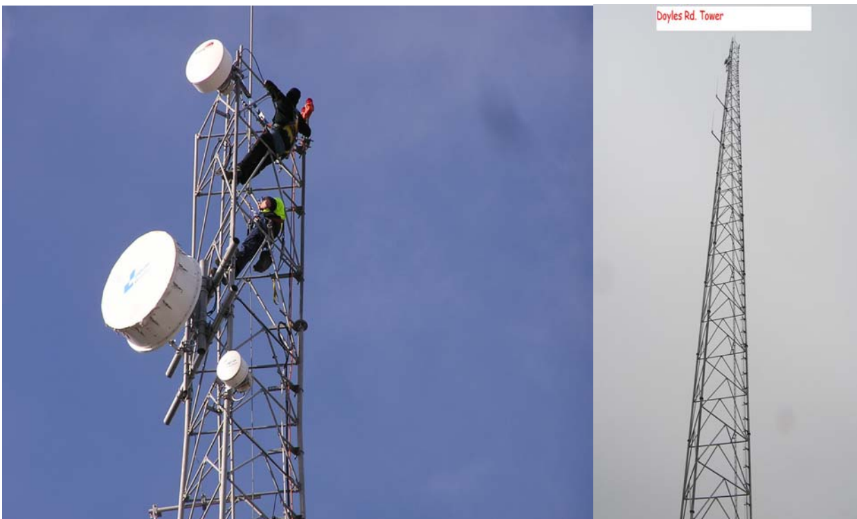
Wave1 Engineers and Riggers working at Doyle Tower (Repeater) in Shepparton
