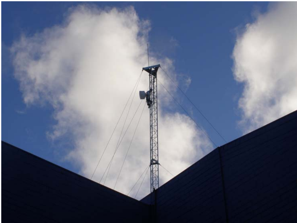
15m mast on top of the SOS Print & Media Head Office
