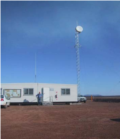
Moorvale Mast & Antenna
